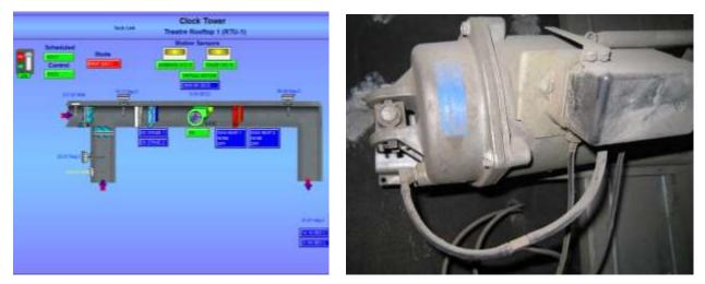
Figure 2.6: Theatre Rooftop Unit – DDC Graphic & compressed air damper actuator
