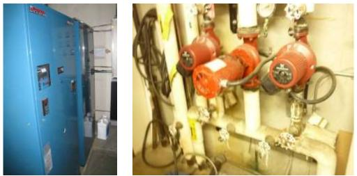
Figure 2.5: Hot water boilers and hot water distribution pumps
