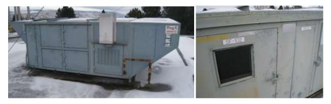
Figure 2.4: Makeup Air Unit & Air Handling Unit (SF-102)
