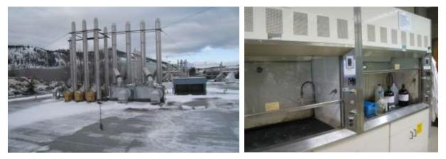
Figure 2.6: Lab Exhaust Fans and Fume Hoods
