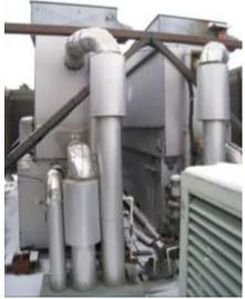
Figure 2.10: Fluid Cooler(s) located on roof
