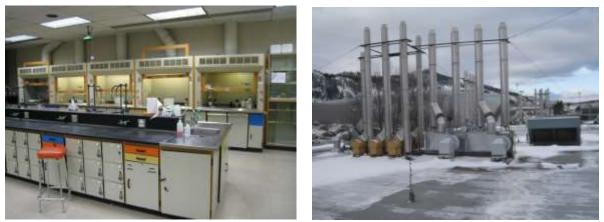
Figure 10: Fume hood exhaust and fans
