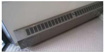
Figure 2.8: Wallfin Convectors in Stairwells
