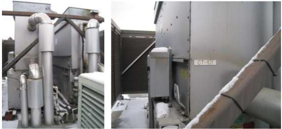
Figure 11: Cooling Towers located on the building roof
